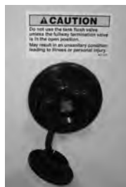
Tank Flush Inlet
